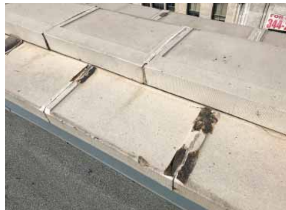
Woolworth Building. Terra cotta parapet at the north facade, with failed sealant at many joints between units. JGWA, 2019.
