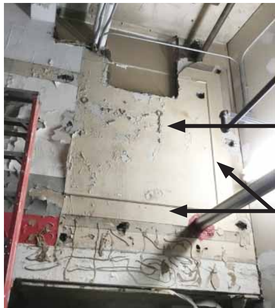
Woolworth Building. Evidence of the historic lunch counter remains in the southwest corner of the first floor. The doorway in the south wall (upper right image) led to the kitchen. The lunch counter area retains remnants of the historic wall treatment, with painted plaster walls surfaces, applied wood trim to create "panels", and composition swag (lower right image). The outline of the counter can be seen on the floor (lower left image). The red tiled area marks the serving area inside of the counter. Round holes along the perimeter of the counter show the location of the stools. JGWA, 2019.
