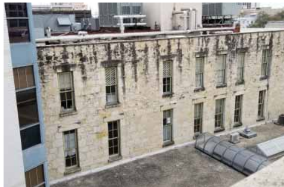
Crockett Block. West elevation. Note the staining at the top of the stone wall. JGWA, 2019.
