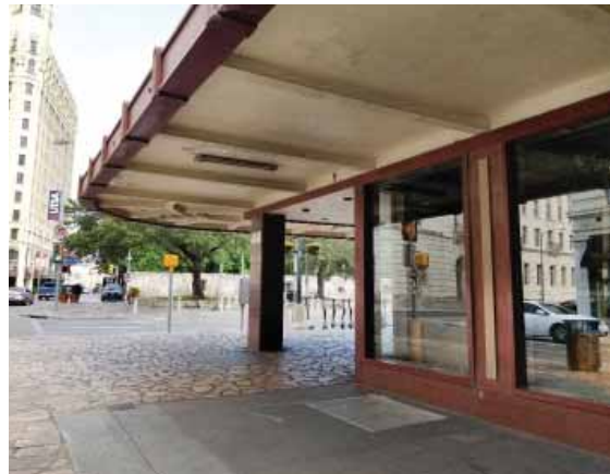
Woolworth Building. Historic canopy at the northeast corner. The concrete patch in the sidewalk is the location of a historic glazed vault light that provided illumination into the basement. The free-standing column was historically clad in terra cotta. JGWA, 2019.
