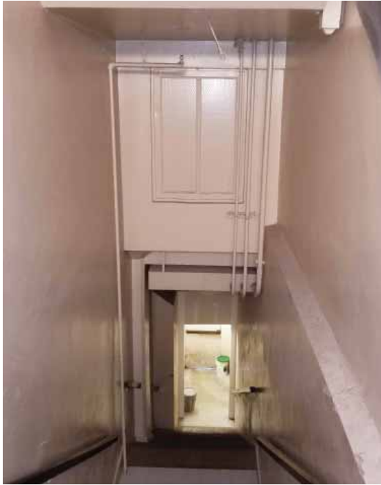
Woolworth Building. Original northwest stair, looking down towards first floor. Note the painted original interior window, which would have provided borrowed daylight from the second-floor spaces into the stairway. JGWA, 2019.
