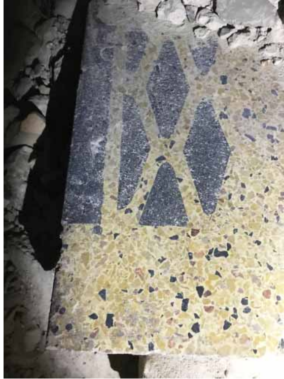
Woolworth Building. Historic terrazzo stair tread detail, at the stairway from the basement to the first floor at the southeast corner of the building. JGWA, 2019.
