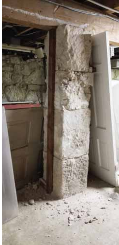
Crockett Block. Basement hallway, looking south (above); and deteriorated stone pier supporting first-floor framing (left). JGWA, 2019.
