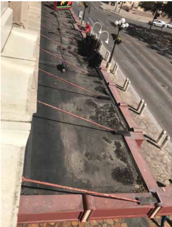
Woolworth Building. Looking north down at the structural support rods and roof surface of the historic canopy over the sidewalk. JGWA, 2019.
