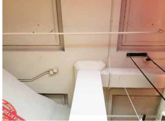
Woolworth Building. First-floor concrete pier with applied profiled wood trim, supporting the coffered plaster ceiling. JGWA, 2019.
