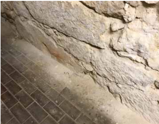
Crockett Block. Deteriorated stone wall in basement, indicating a problem with rising damp. JGWA, 2019.
