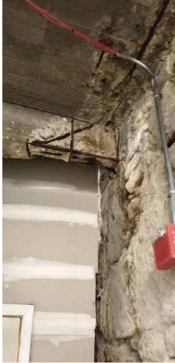
Woolworth Building. Structural deterioration of the reinforced concrete beam at the northwest corner of the basement, below the sidewalk above. JGWA, 2019.
