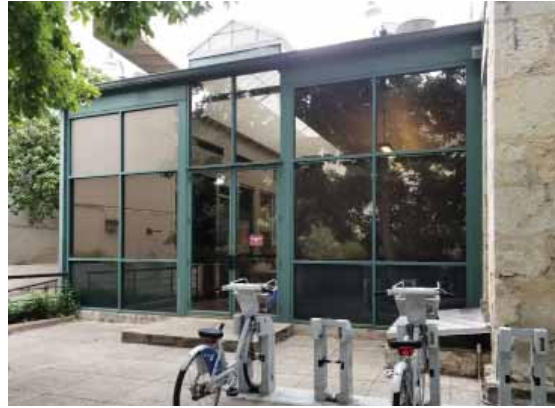
Crockett Block. South entrance to the rear (west) addition, constructed during the 1983 renovations. This one-story metal and glass addition is a non-contributing feature of the building's exterior. JGWA, 2019.
