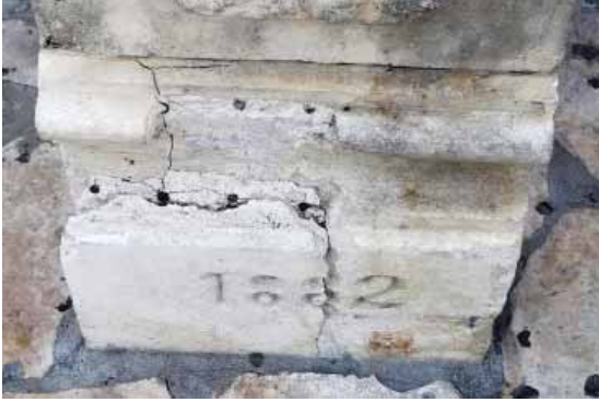
Crockett Block. Deteriorated base of stone pier on east elevation. JGWA, 2019.
