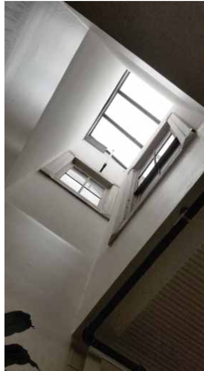
Crockett Block. Existing lightwell, looking up from a second-floor office. Interior windows at the third floor are character-defining features that provided daylight into the central spaces of the buildings. JGWA, 2019.
