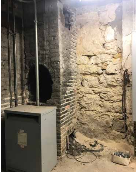
Woolworth Building. Main chimney stack against the west wall. It is possible that the stone foundation wall survives from the Maverick Building, which was demolished for the construction of the Woolworth Building. JGWA, 2019.
